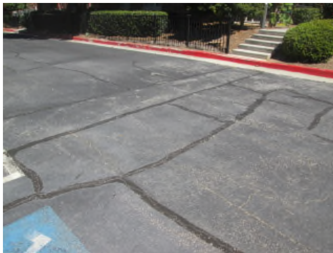
Repairs+crack filling+seal-coat+striping+curb painting
